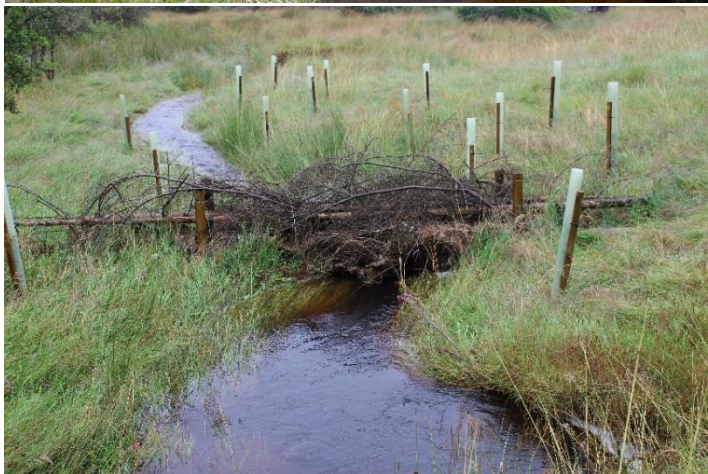
Leaky dams in the Eddleston catchment, Scotland. Credit: Tweed Forum.
