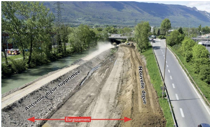
Figure 5. Construction works: setting back the levee.
