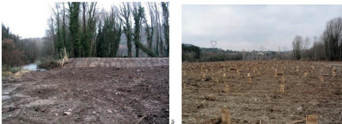
Figure 9. On the left, the newly constructed levee delineates the area. On the right, 5000 trees are planted in the area to decrease flow velocity during floods. Source: Syndicat intercommunal d'aménagement hydraulique des bassins de la Clamoux, de l'Orbiel et du Trapel (SBCOT)
