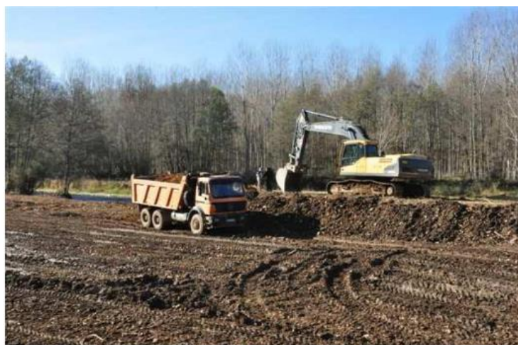
Figure 3. An artificial levee is lowered to recover lateral connectivity.
