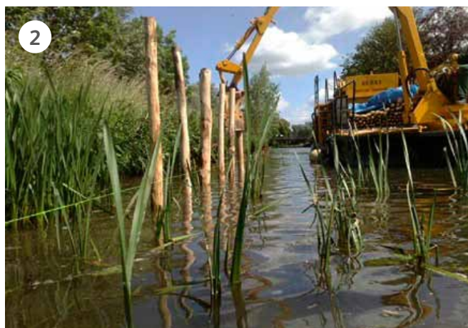
(1) Survey line for position of retaining posts for coir rolls. Shows extent of erosion and lack of marginal vegetation; (2) Pile driving posts
