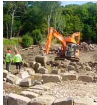
(1) View downstream during construction; (2) Installing tombstones to low stone weirs
