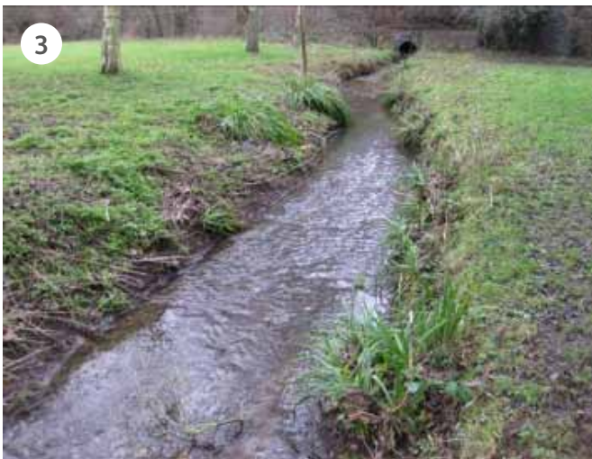
(3) Current soft-engineered channel, with new sinuosity resulting in (4) increased morphological diversity and natural erosion and deposition patterns
