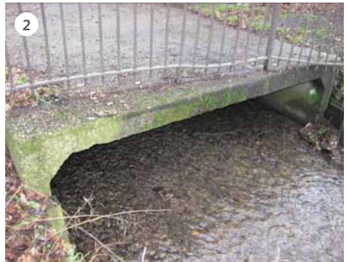
(1) Previous toe-boarding of straight channel and (2) concrete bridge from 1950 / 1960s channelisation;
