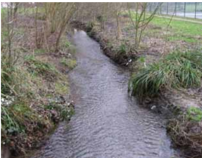
New, restored channel
