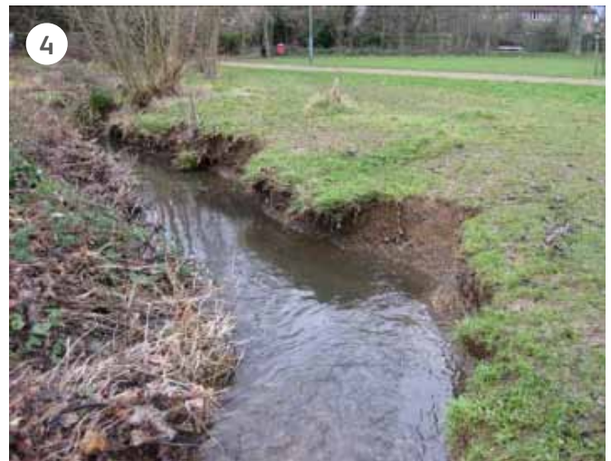
(3) Current soft-engineered channel, with new sinuosity resulting in (4) increased morphological diversity and natural erosion and deposition patterns
