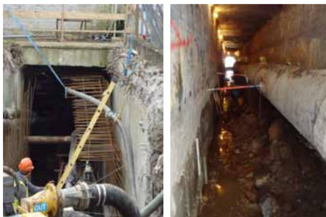
Poundstreecher culvert during refurbishment works still showing services within culvert
