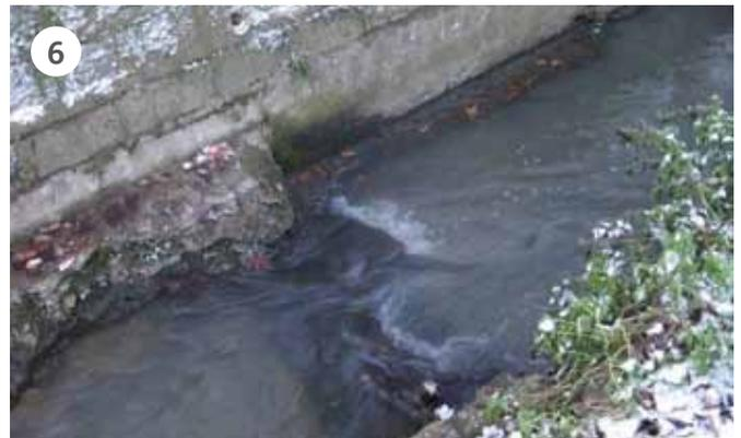
(1) Reach where toe-boarding has been removed; (2) pine-box deflectors backfilled with gravel; (3) small flow deflectors; (4) artificial riffle in a straightened section of the channel; (5) remeandering of previously straightened channel; (6) former location of weir with concrete base and banks retained.
