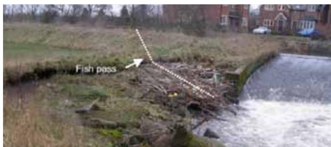
A 1.8 m wide Larinier Superactive baffle fish pass was constructed to enable fish passage over Heatley Weir, requiring two flights with an intermediate resting pool. The fish pass was located immediately below the weir on the right bank, and the fish pass routed across the flood plain, as shown above. The length of each flight is approximately 8.8 m at a gradient of 15 %, with retaining walls high enough to prevent the ingress of flood waters.
