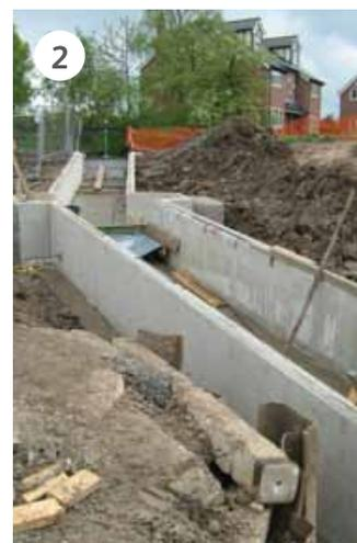
(1) Concrete U-channel of the fish pass during construction;
