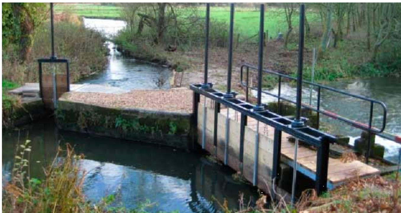
**Hyford Hatches: restored allowing more effective and safe water level management through operation control.**
