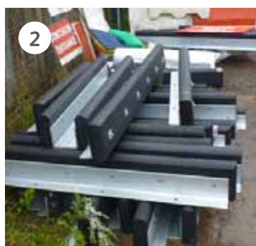
(1) Plan of baffles on downstream weir face (crest of weir at top of diagram); (2) Baffles prior to construction
