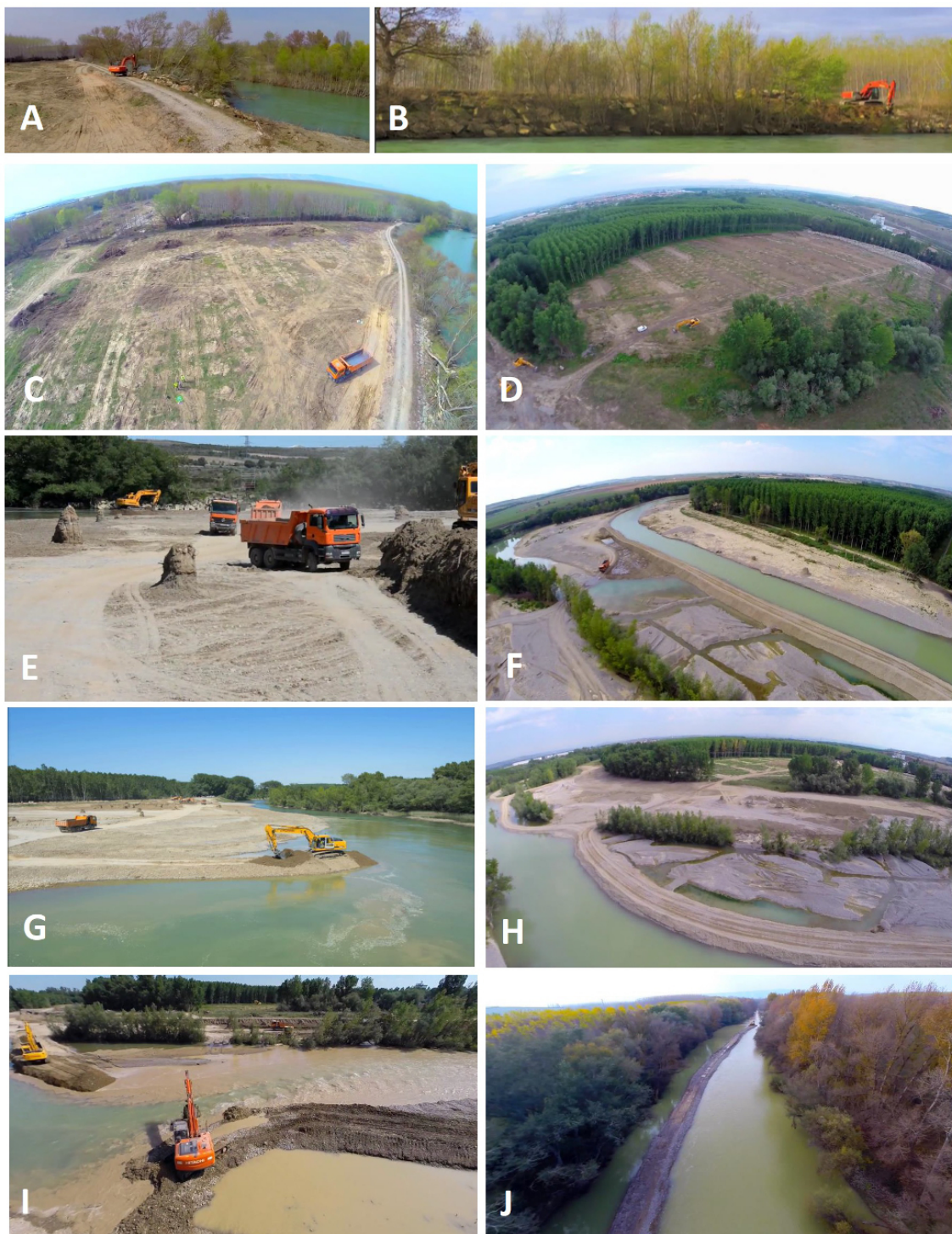
Restoration process: Removal of dykes (B); suppression of ripraps (A); recovering riparian space (C, D); recovering space for beds and widening the main channel (E, F, G); returning to the river the sediments dredged during the past (H, I, J).
