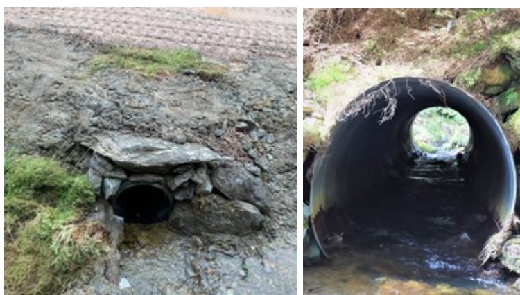
Figure 8. Sediment traps and culvert improvements
