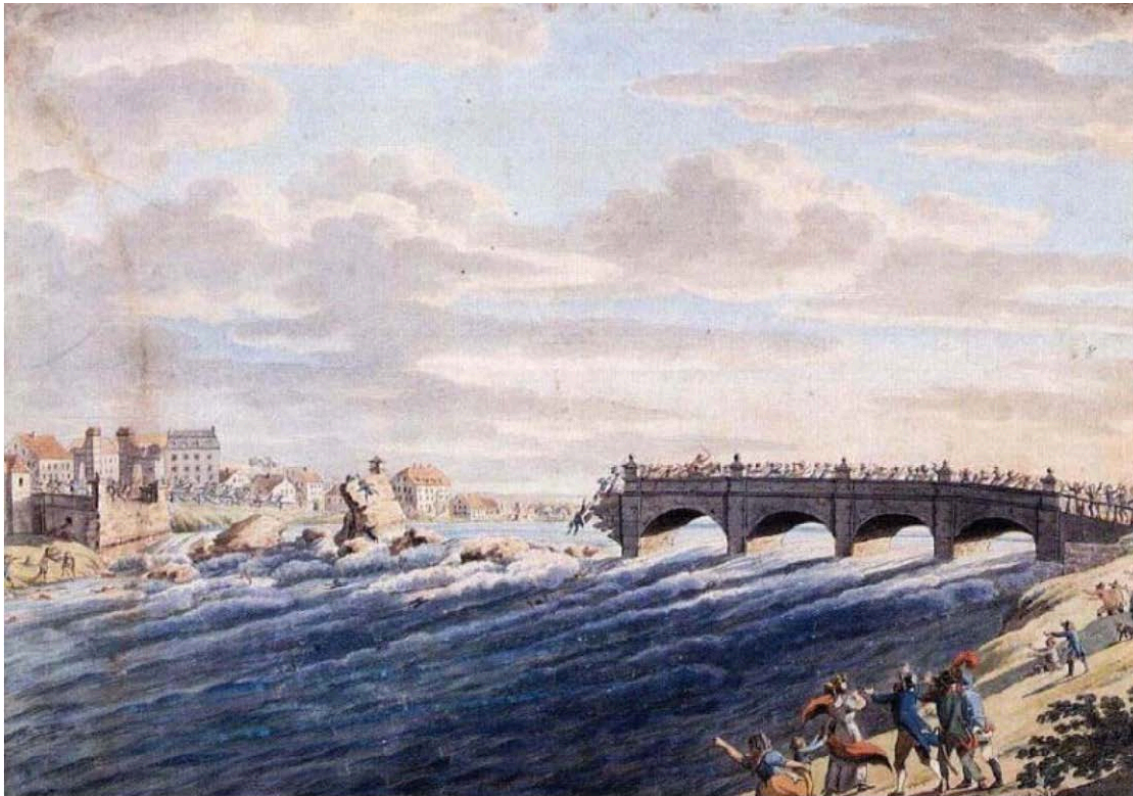
Figure 4. Destruction of Ludwigs Bridge in 1813 (Sopena, 2013)
