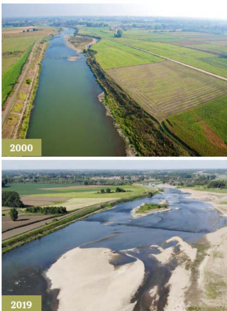
Figure 4. Before and after the widening of the river channel (Source: maasinbeeld.nl).
