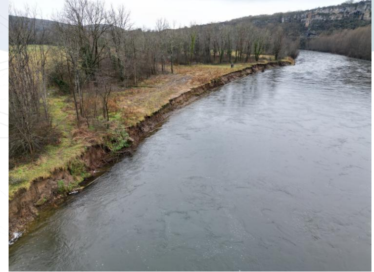
Removal of a riprap in Floirac – February, 2025
